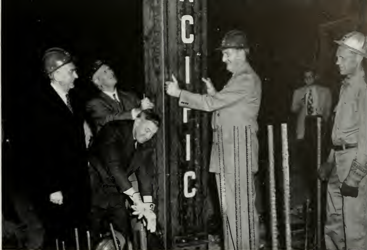
Laying the cornerstone of UCLA's new medical building in the modern way, Regent EDWARD DICKSON bolted the first rivet as, left to right, President SPROUL, Governor WARREN and Med School dean, STAFFORD L. WARREN, stood by. With years of planning about to become a reality, the dedication ceremonies were a milestone event in the history of UCLA.
